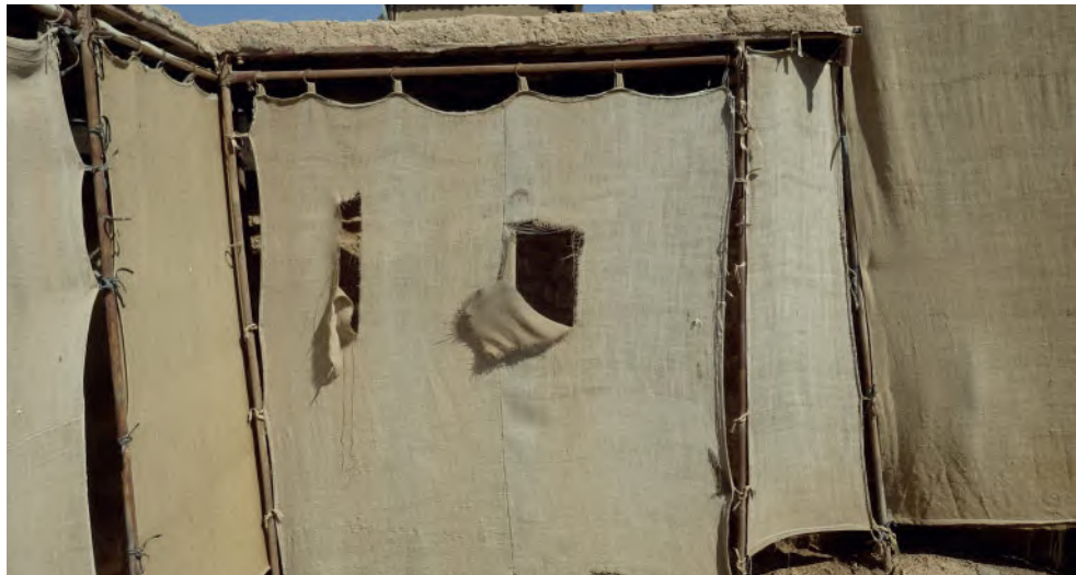
Holes in the curtains caused by rain, wind and birds
