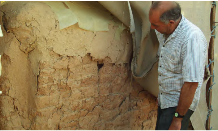
Mohammed Omo inspecting a mud brick wall
