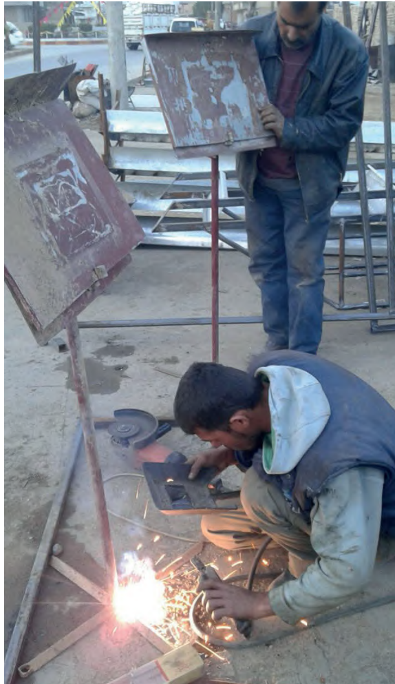
Repair work of one of the reading stands: welding the metal structure and repainting
