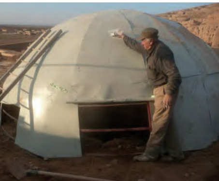
The new "dome" completed, with openings at the base
