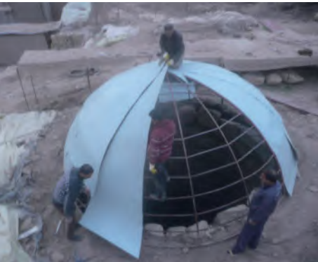
Working on making a new metal cover
