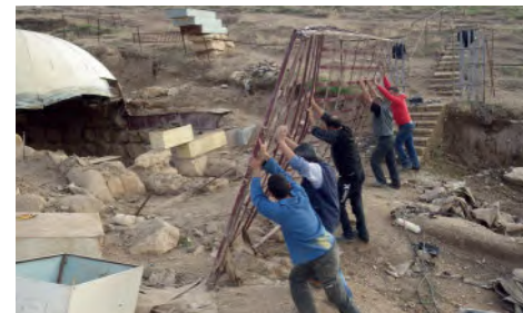
Painting the entire metal cover in 2016, and new metal cover of the Abi entrance
