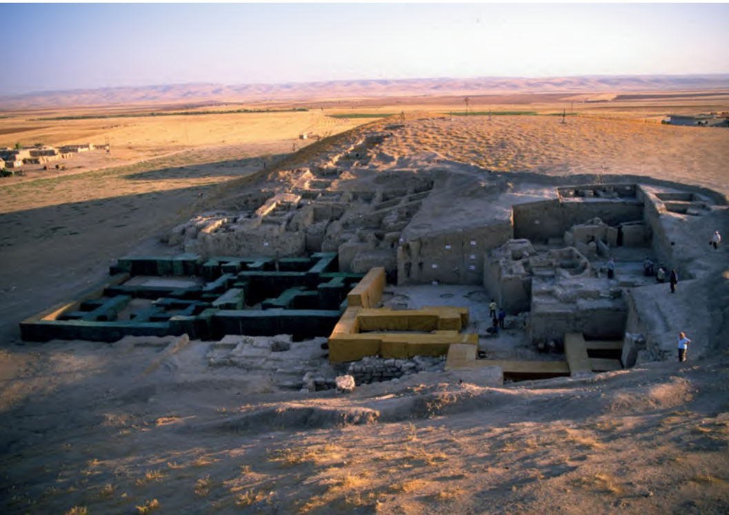
The Urkesh Palace with the protective system for the mud brick walls (2250 B. C.)
