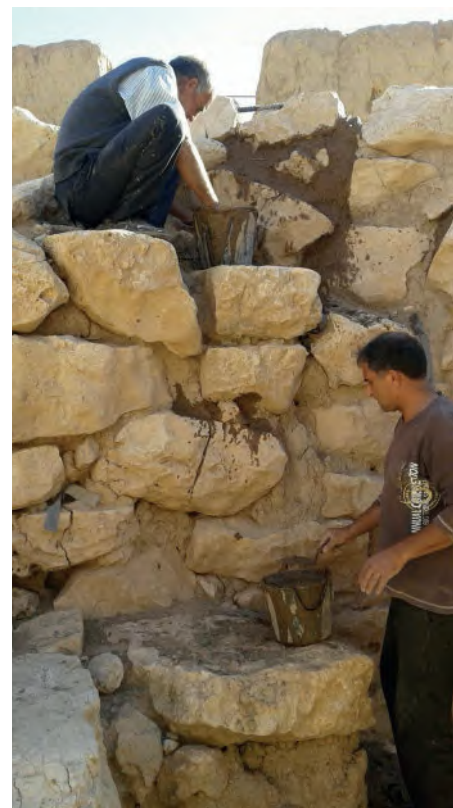
Refilling the mud between the stones of the Temple Terrace wall
