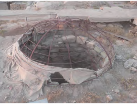
The Abi and its burlap cover, completely destroyed by the wind (2013)
